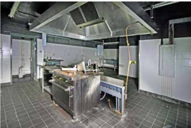
The kitchen still contains much of its stainless steel equipment
